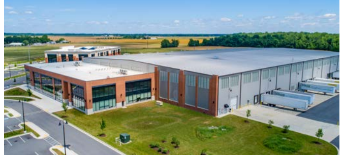
Distribution Center: Chestertown, Maryland
