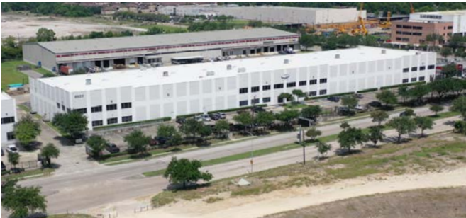
Distribution Center and Manufacturing: Houston, TX
