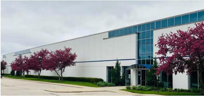
Dixon Sanitary: Pewaukee, Wisconsin
